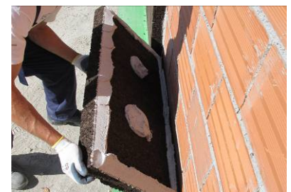
3. Placing the panel on the support
