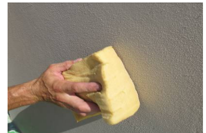
16. Sponging the surface to obtain smooth sanded finish
