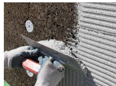
11. First spreading of ADHERE Vit ecoCORK
