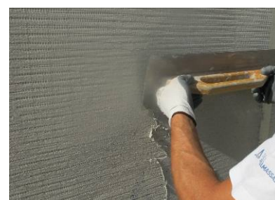
13. Second spreading of ADHERE Vit ecoCORK
