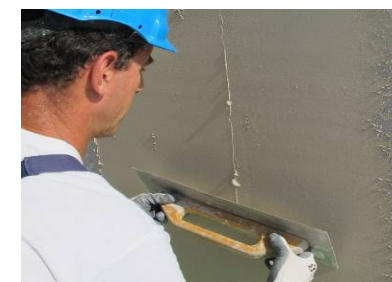
14. Application of first layer of REABILITA Cal Acabamento (Finish)
