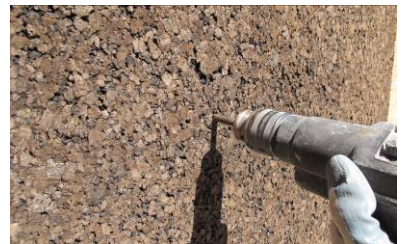
7. Drilling holes for putting mechanical fixing
