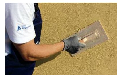
19. Application of acrylic finish REVDUR
