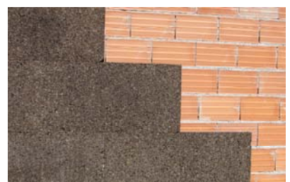
5. Placing the panels by rows
