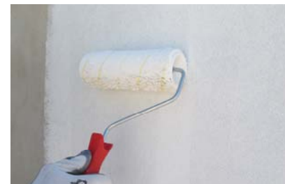
17. Application of SecilTEK SP 01 on SecilTEK AD 25
