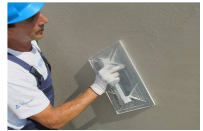
15. Trowelling of final surface of REABILITA CAL Acabamento
