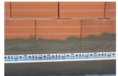
1. Fixing startup profile and support waterproofing.
