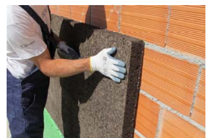
4. Fixing the panel by pressing it
